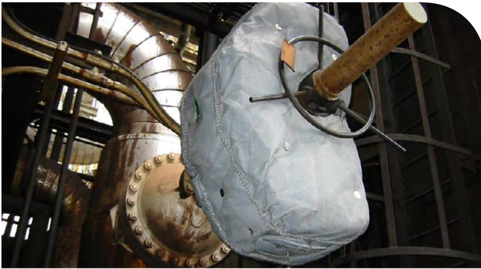
VALVE ACTUATOR ENCLOSURE Design: FB2000MSSiSiM - 3.5" Thickness
