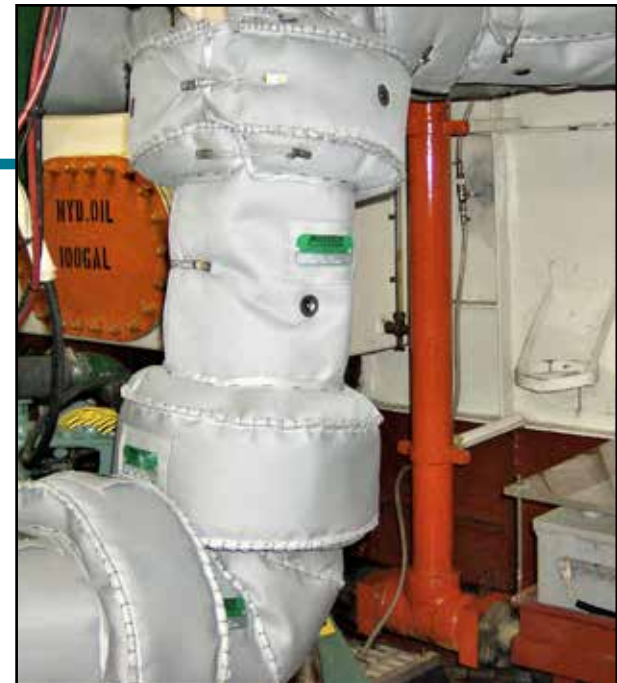
MT850SGM ENG EXHAUST PIPING, ELBOWS, FLANGES & EXP JOINTS
