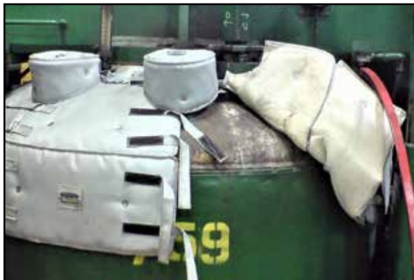
MT800SGM REMOVABLE REUSABLE BLANKET INSULATION
